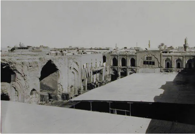
Figure 1. The courtyard of the madrasa Mustanşiriyya before restoration. Copyright of https://www.archnet.org/sites/3836
